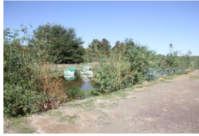
One of the two unlined Primary Ponds
