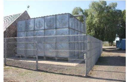
Steenrots Storage Tank 0.104 ML
