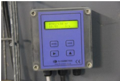
Reclamation Plant: Final flow display unit
