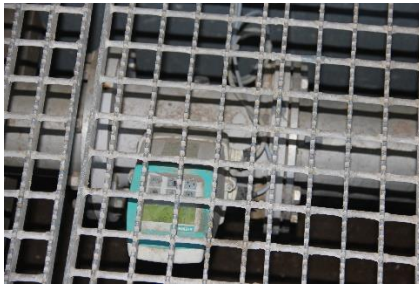
Reclamation Plant: UV feed flow meter
