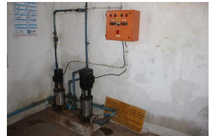
Disinfection pumps (Chlorine gas)
