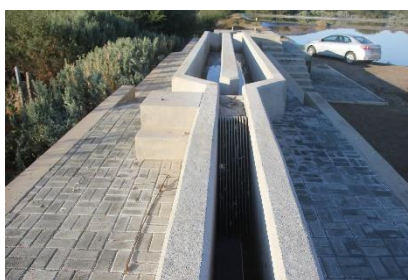
Inlet Structure with grit channels
