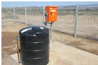
Disinfection at Moddergat Borehole (Sodium Hypochlorite)
