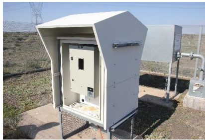
Steenrotsfontein SR10 (Scada system vandalised)
