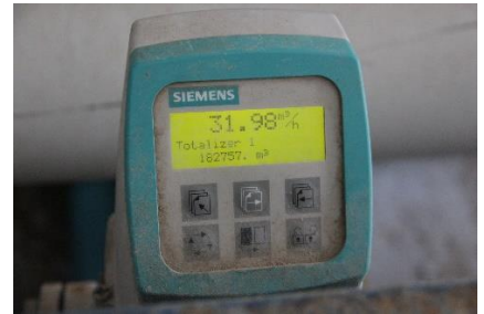
Reclamation Plant: Waste flow meter
