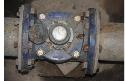
Inlet of WTW (150mm)
