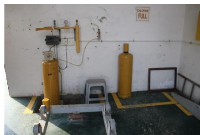
Disinfection (Chlorine gas)
