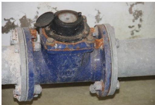
Murraysburg WWTW: Final effluent irrigation meter
