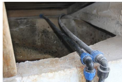
Aluminium Sulphate dosing
