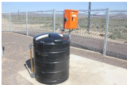
Disinfection at Riverside Borehole (Sodium Hypochlorite)
