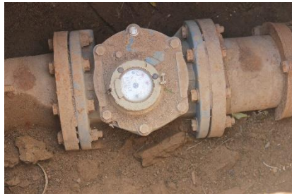
Outlet of WTW (150mm)
