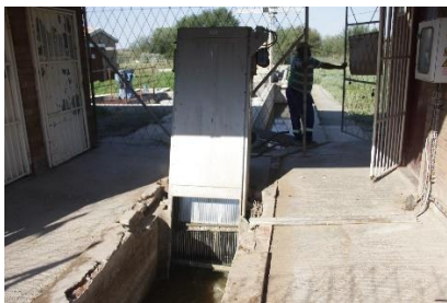
Inlet Structure (Mechanical screen)
