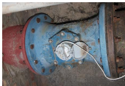
Bulk supply to town (300mm) at reservoirs
