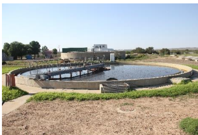
Secondary Settling Tank
