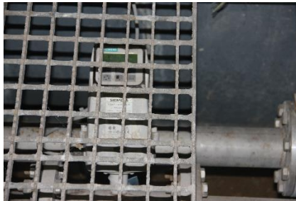
Reclamation Plant: RO feed flow meter
