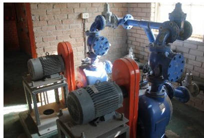
Sludge Pumps (Only one operational)
